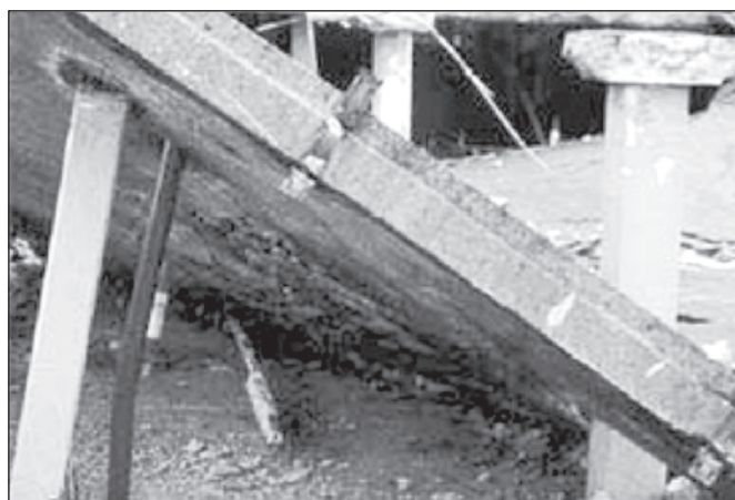
d) Piper Rows Car Park, 1997 Autor: Woods [5]
